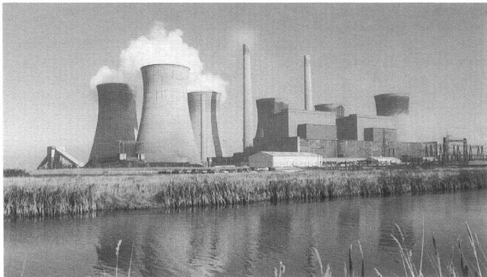
Figure 13.14. Natural draught water-cooling towers
